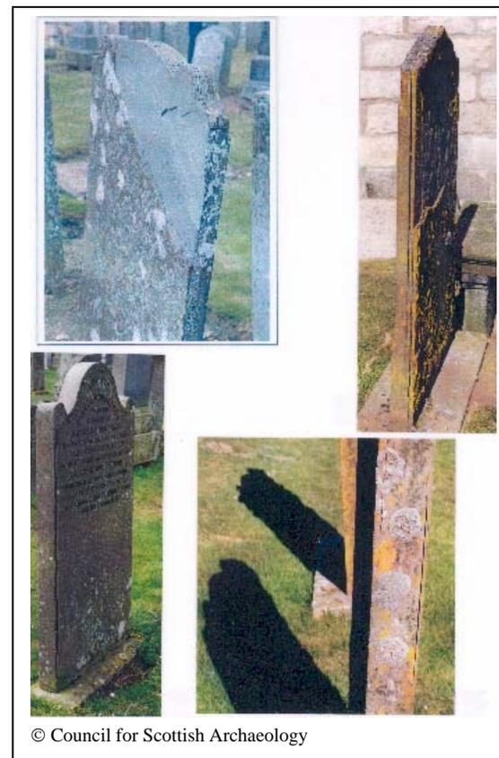
**Planar erosion** is material loss whereby layers of stone become detached from a stone's surface. There are four types of planar decay
