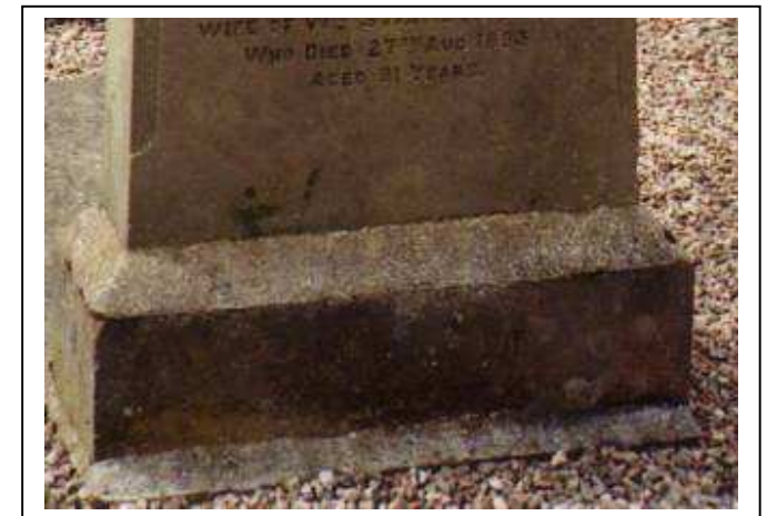
Figure 59 Gravestone repair using concrete
