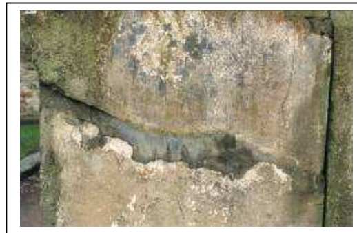
Figure 58 Repair using a cement mortar
