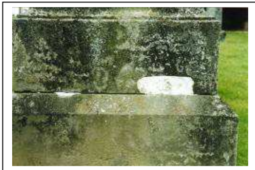
Figure 57 Lime mortar plug
