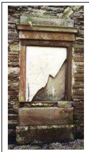
Figure 45 Broken marble panel in sandstone surround
