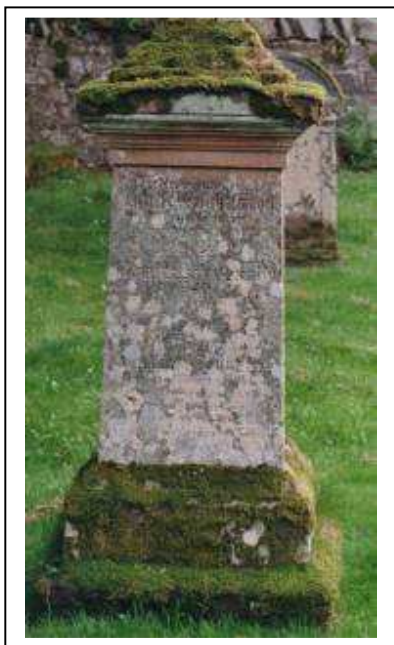
Figure 62 Extent of moss growth here, to the upper and lower thirds of the gravestone is major
