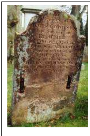
Figure 53 Headstone with iron clamps
