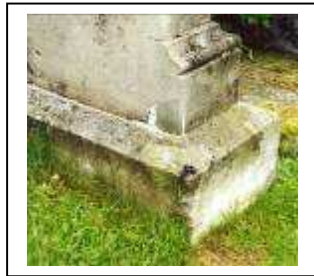
Figure 55 Stone repair fixed with lime mortar
