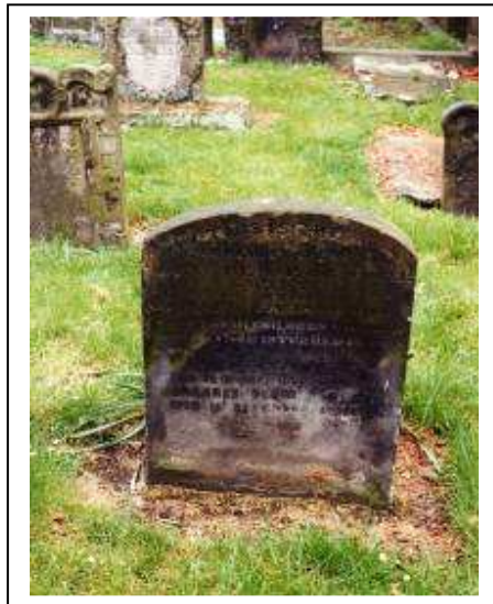
Figure 66 Grass killer used around headstone in foreground. Flat stone in the background covered with grass-cuttings.
