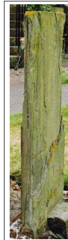
Figure 76 Major contour scaling on carved surface
